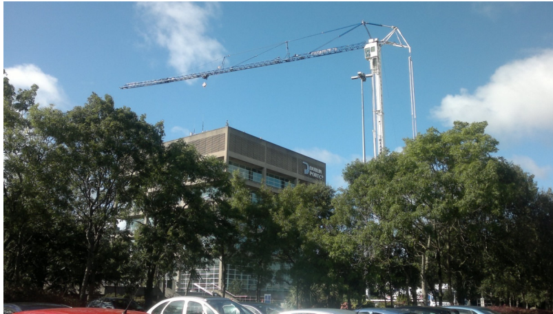
Crane lifts new boilers and microCHP to rooftop boiler house
